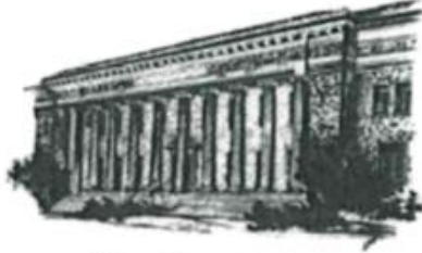
Tehama County Courthouse
